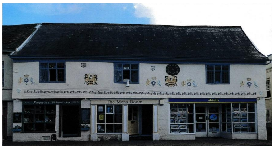
Fig: 13. 46-48, High Street at Hadleigh, Suffolk. A building with heraldic devices executed in pargetting: including the arms of the Bayning family.
