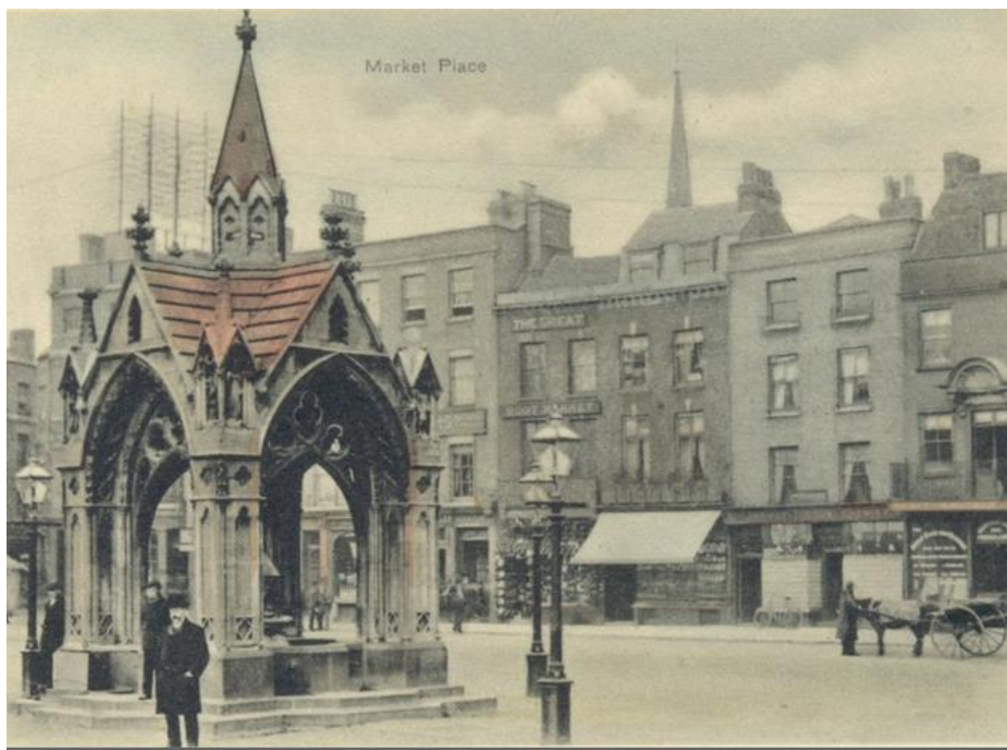
Figs: 5 & 6 Market Place Fountain. Erected 1855 – Demolished 1953. The base remains in the Market Place. The Town Council had allowed the structure to fall into a state of disrepair.
